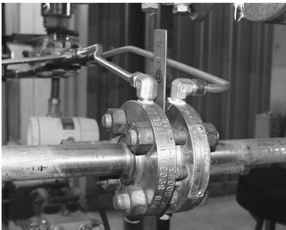
FIGURE 9.7 Orifice plate flow meter.
